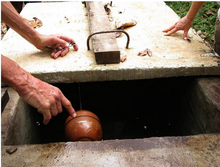
Float valve in break-pressure tank, Bajo Cacicon
