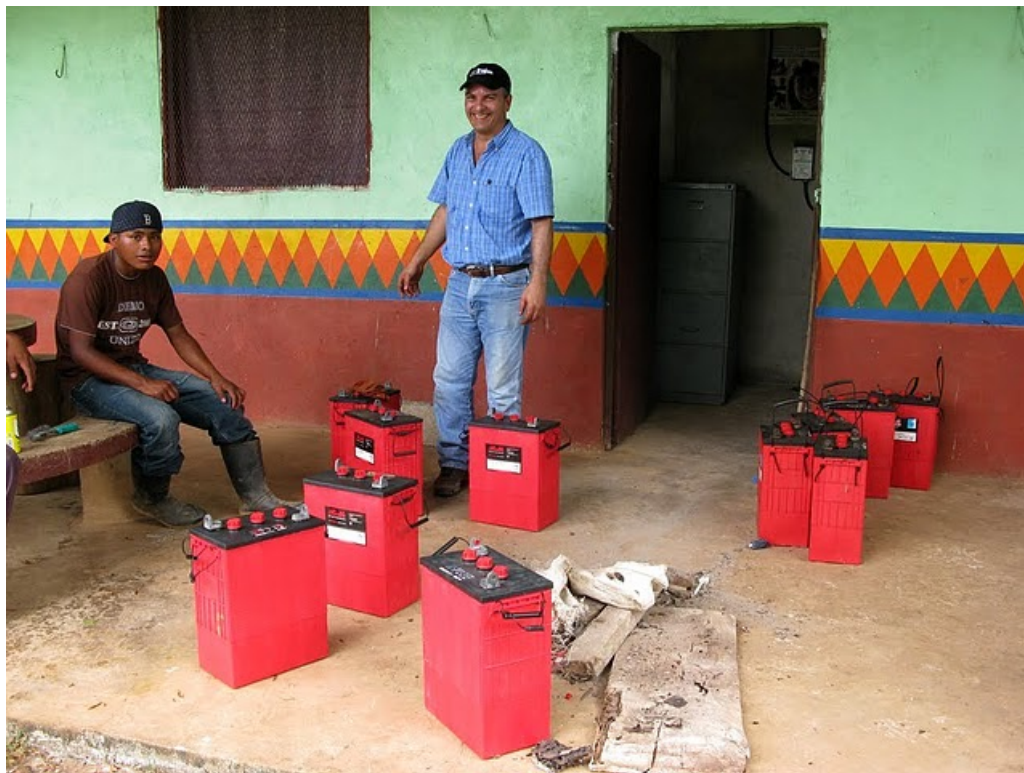
Victor and assistant changing out batteries for the photovoltaic system, Llano Ñopo
