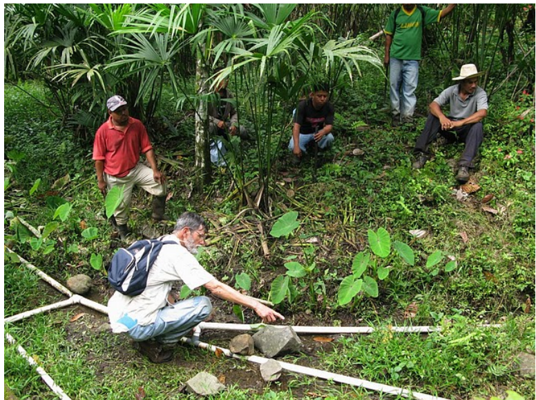
Examining piping at Limon toma
