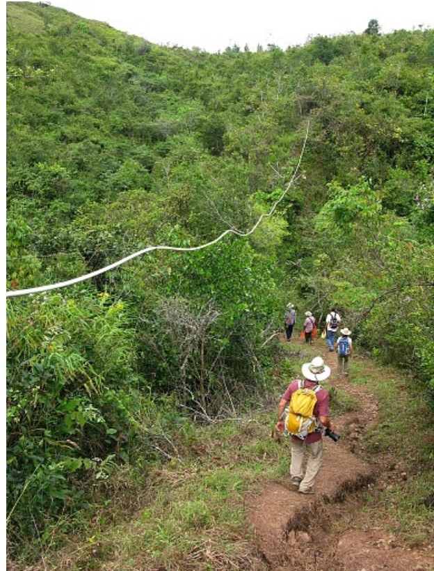
Suspension pipe crossing, Changoso
