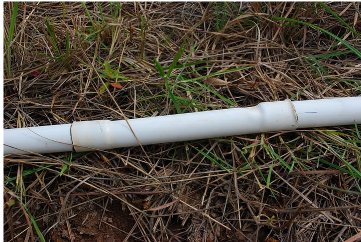
Pipe coupler formed from salvaged tubing
