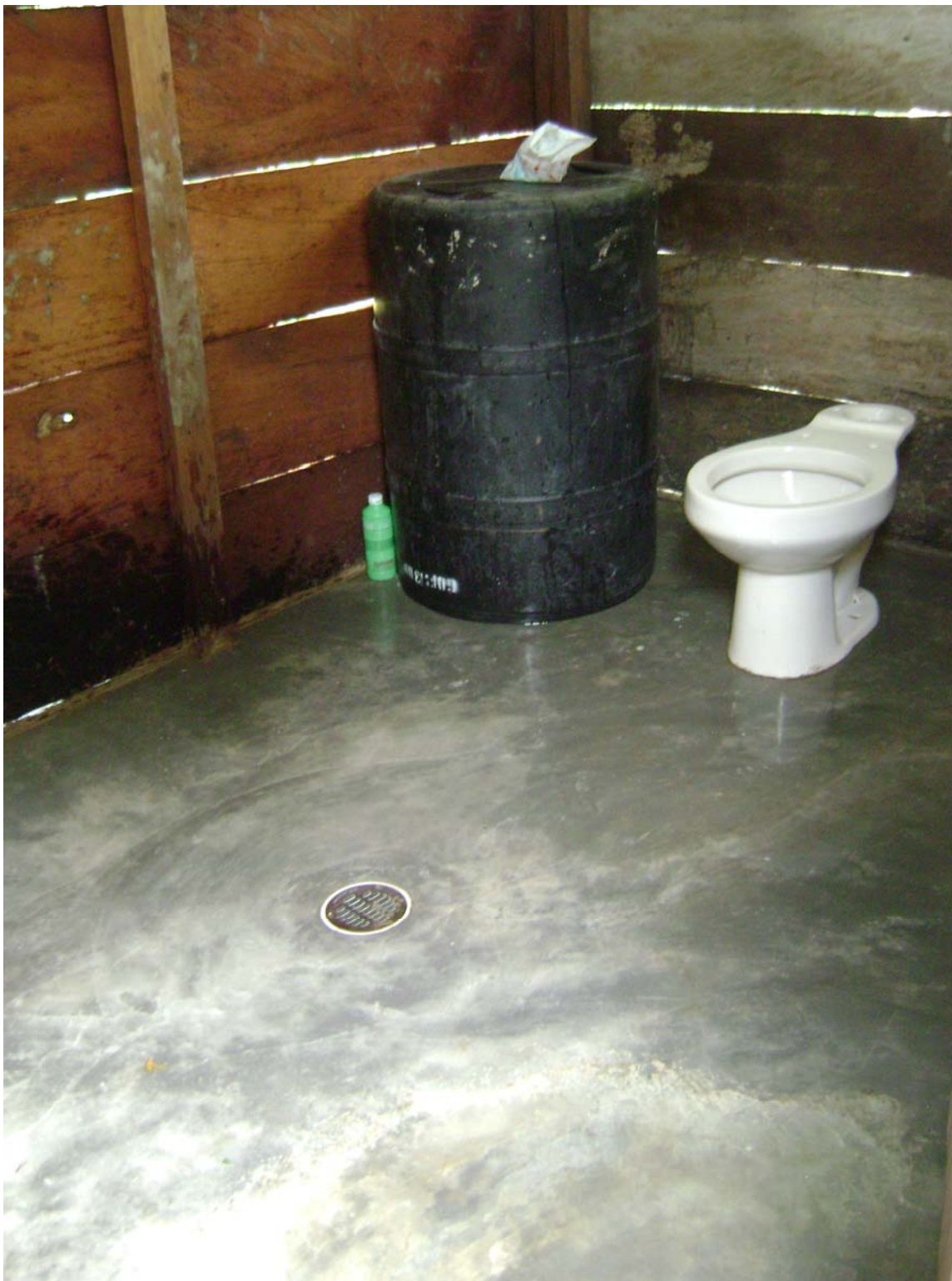
Example of Interior Latrine Construction
