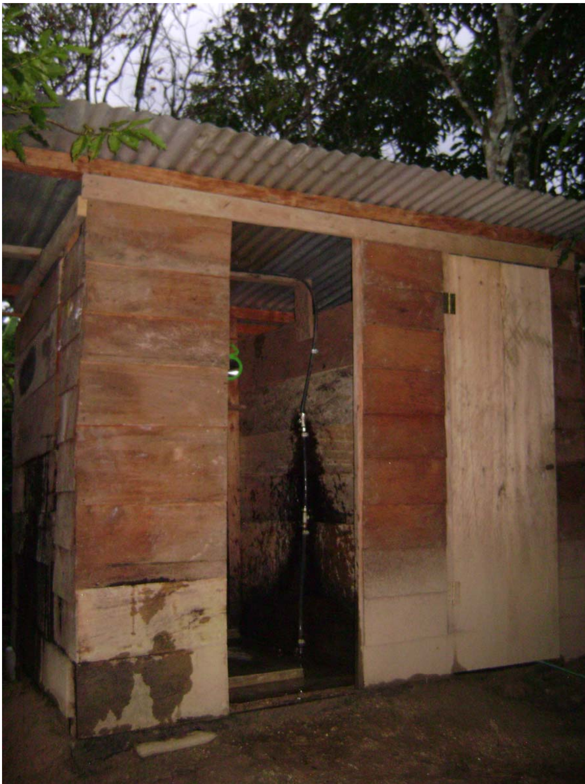
Example of Exterior Latrine and Shower Construction
