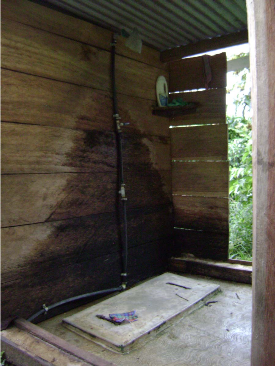
Example of Interior Shower Construction
