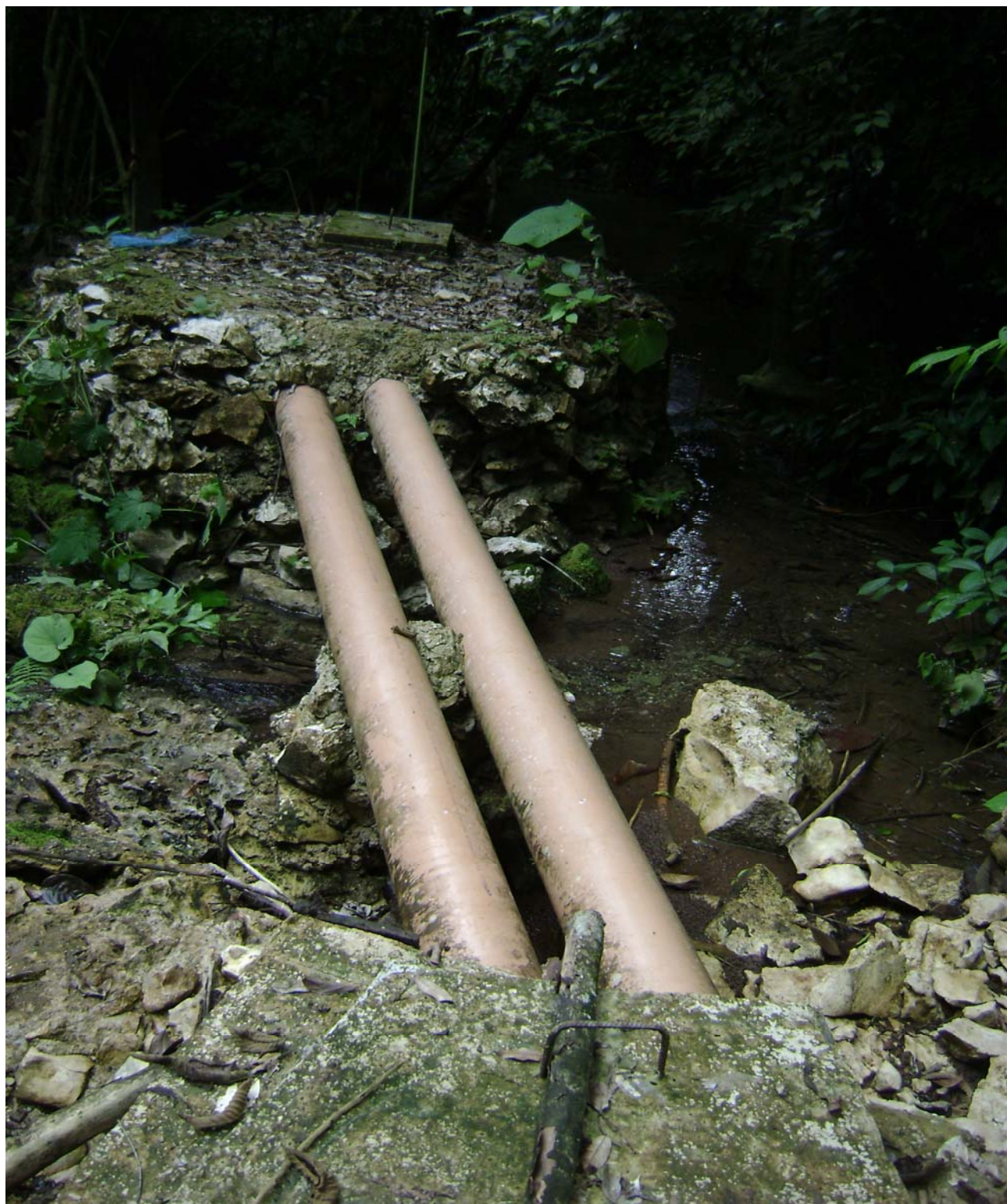
Laguna Chum Cerro Spring Catchment System Post Construction
