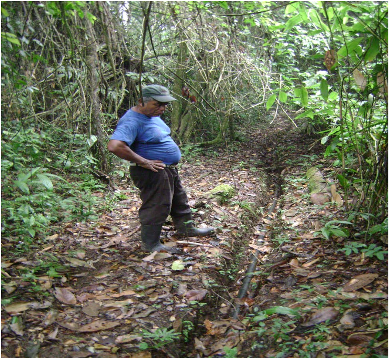
Lazaro examines location where trench needs to be 50 cm deeper to maintain good gravity
